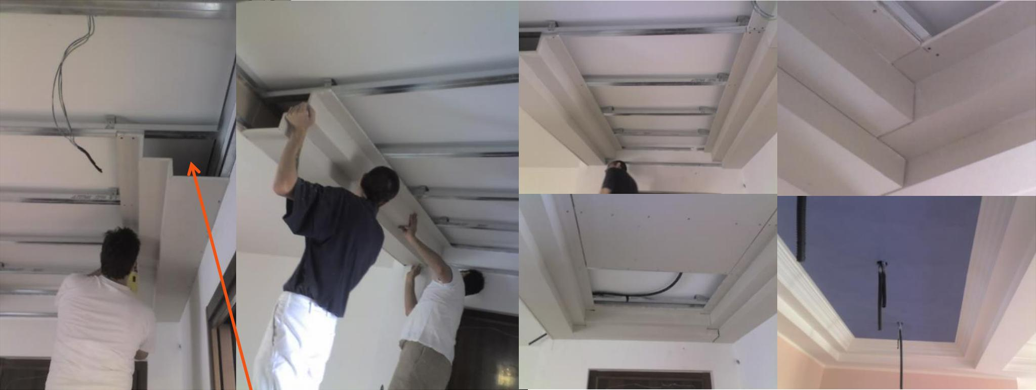
Parts are glued – reduce metal framing and save time!
